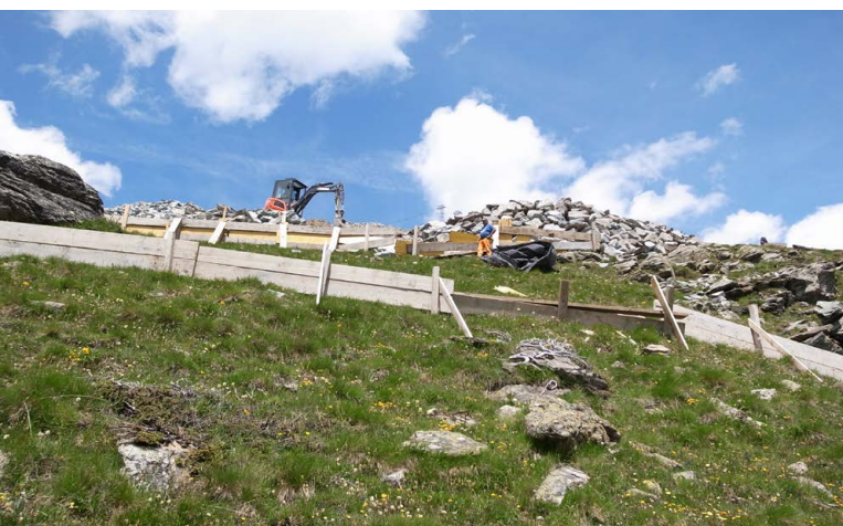
Figure 16: Formwork panels secure the construction site and prevent material from sliding into the areas below [photo: M. Peters].
