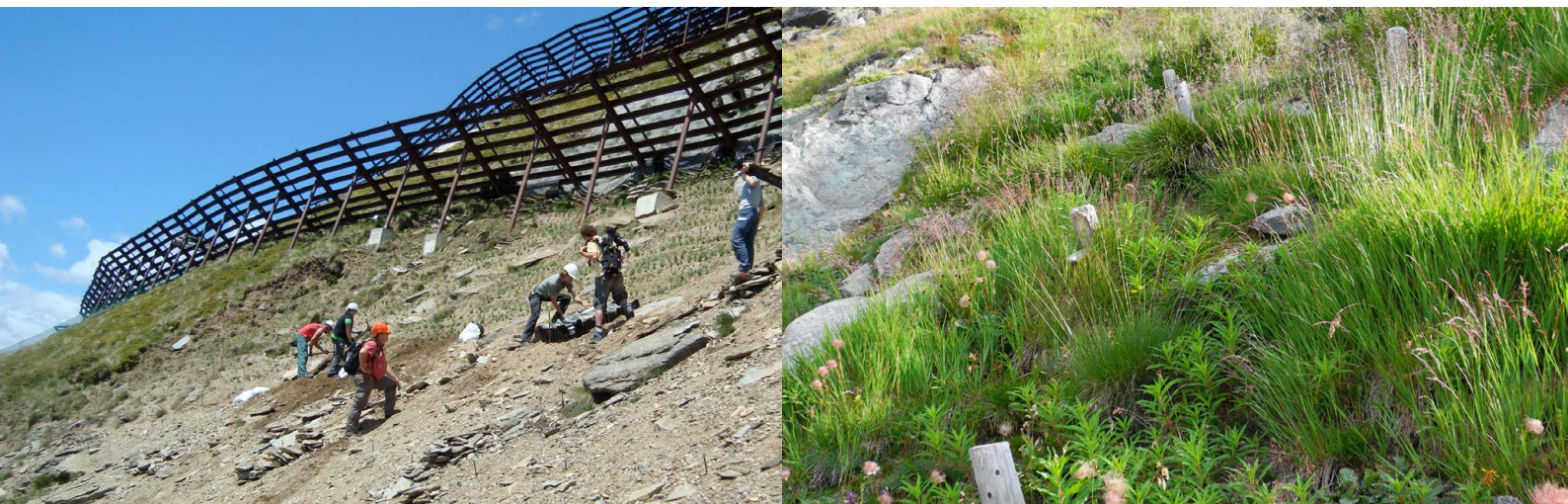
Figure 25: Planting pre-grown seedlings is worthwhile where exposed soil on steep slopes requires stabilisation (Photo: M. Schutz). This approach can result in successful restoration (photo: K. Edelkraut).
