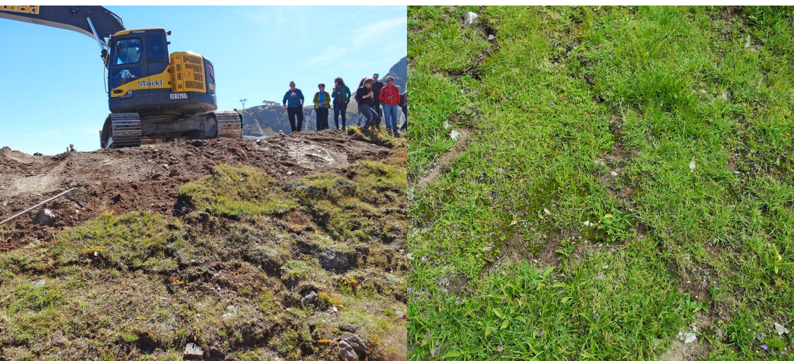
Figure 24: When securing and setting the sods, excavator and manual labor are required [photo: B. Krüsi]. Later, the intervention is often hardly visible or not visible at all [photo: K. Edelkraut].
