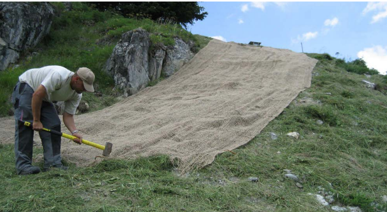
Figure 30: Fastening the geotextiles with wooden nails. Care must be taken to ensure continuous contact with the soil, especially in the case of fine-meshed fabrics and mats [photo: M. Schwager].
