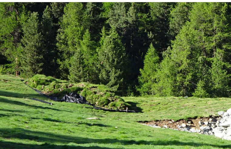
Figure 18: Soil stockpile, covered with sods [photo: K. Edelkraut].
