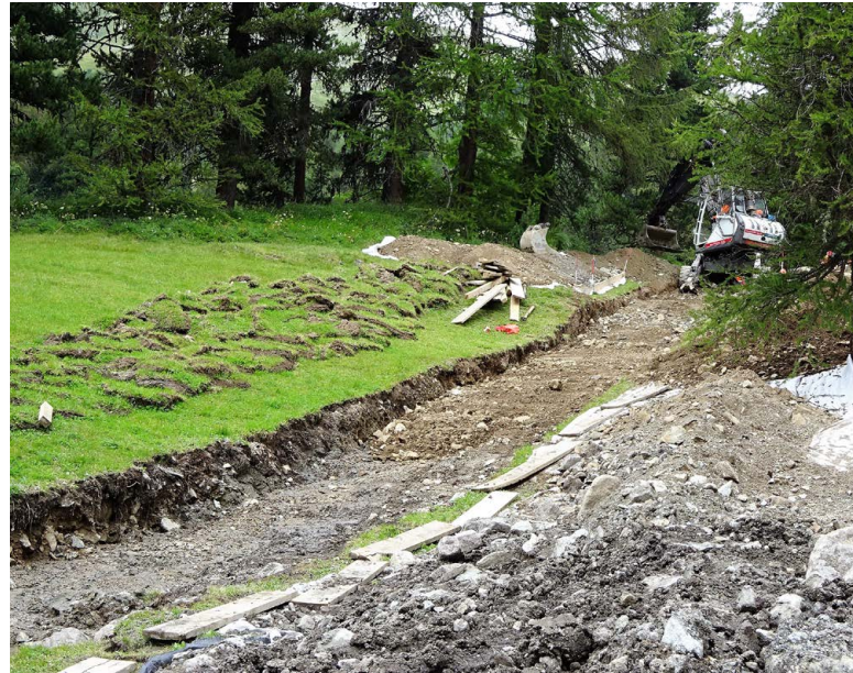
Figure 19: Short-term storage of sod directly on existing vegetation. The soil stockpiles are poured onto a separation layer [Photo: K. Edelkraut].
