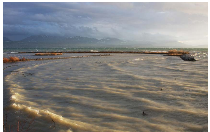
Figure 9: The Bird Island during a storm in 2008. The photo was taken from the shore; the spit is visible on the left, with the riprap embankment directly in front of it. The waves are deformed by diffraction and refraction and spread out in the sheltered area.
