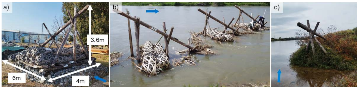
Figure 4: [a] Exemplary Seigyu at Uji-gawa Open Laboratory, Kyoto University; [b] Half-submerged Seigys in Kizu River, Kyoto Prefecture [Kobayashi et al., 2022]; [c] Seigyu in Kizu River seven years after implementation, the blue arrow indicates flow direction.
