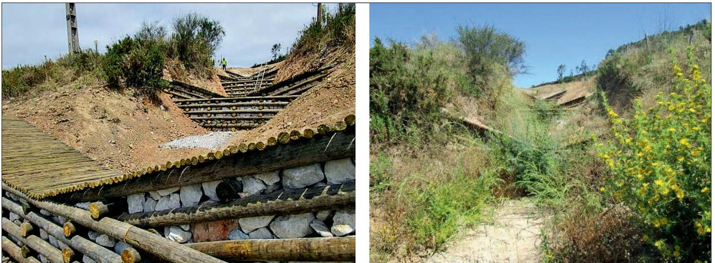
Figure 9: Vegetated wooden weirs after the construction July 2014, and in June 2015.
