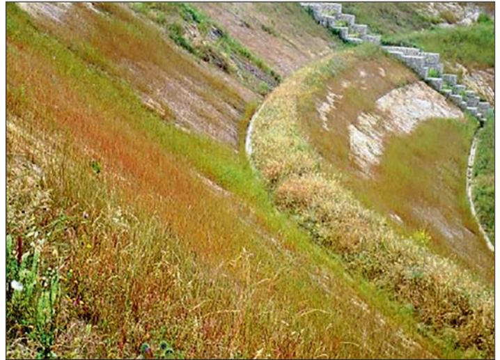
Figure 6: On the left sowings with straw mat, April 2015. On the right herbaceous cover on the slope steps processed with hydroseeding, May 2015; in the right picture slope surfaces not green are rocky arenites, intentionally not processed with hydroseeding.
