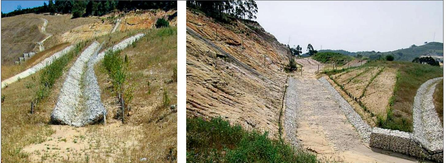
Figure 10: Temporary water runoffs treated with vegetated gabion mats and living combs, June 2015.
