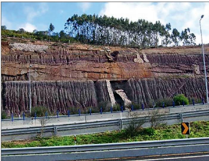
Figure 1: Gully erosions over the entire slope and sliding down ripraps, 2013.
