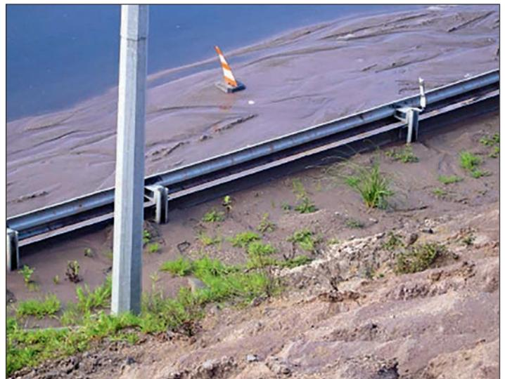
Figure 2: Deposit of fine clay on road surface from silted surface drainage system, 2013.
