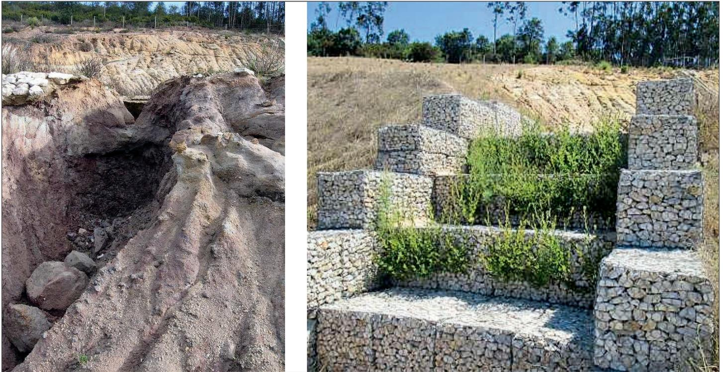
Figure 8: Erosion and mobilization of rocks, 2013; upper vegetated gabions June 2015.
