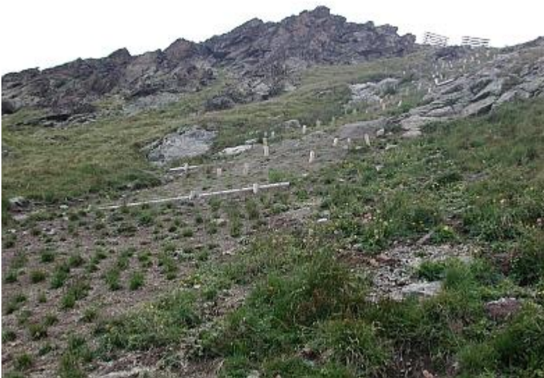
Foto: N. Locher Oberholzer, Working group for high altitude restoration Planting of steep slope, ski world championship 2003, St. Moritz, 2800 m ü. M.
